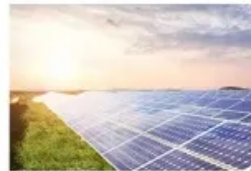
Energy Storage System
