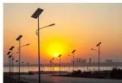
Solar Street Light
